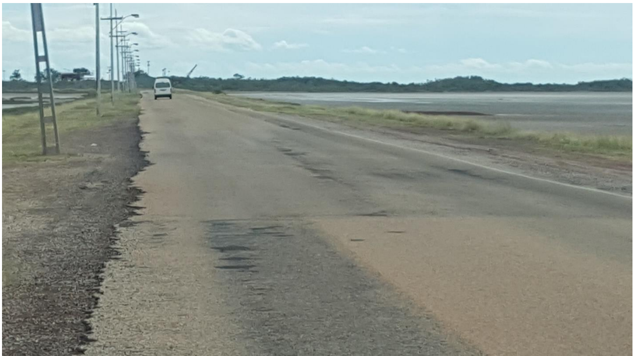
Edge Break, Jetty Rd – Condition 4, Poor
