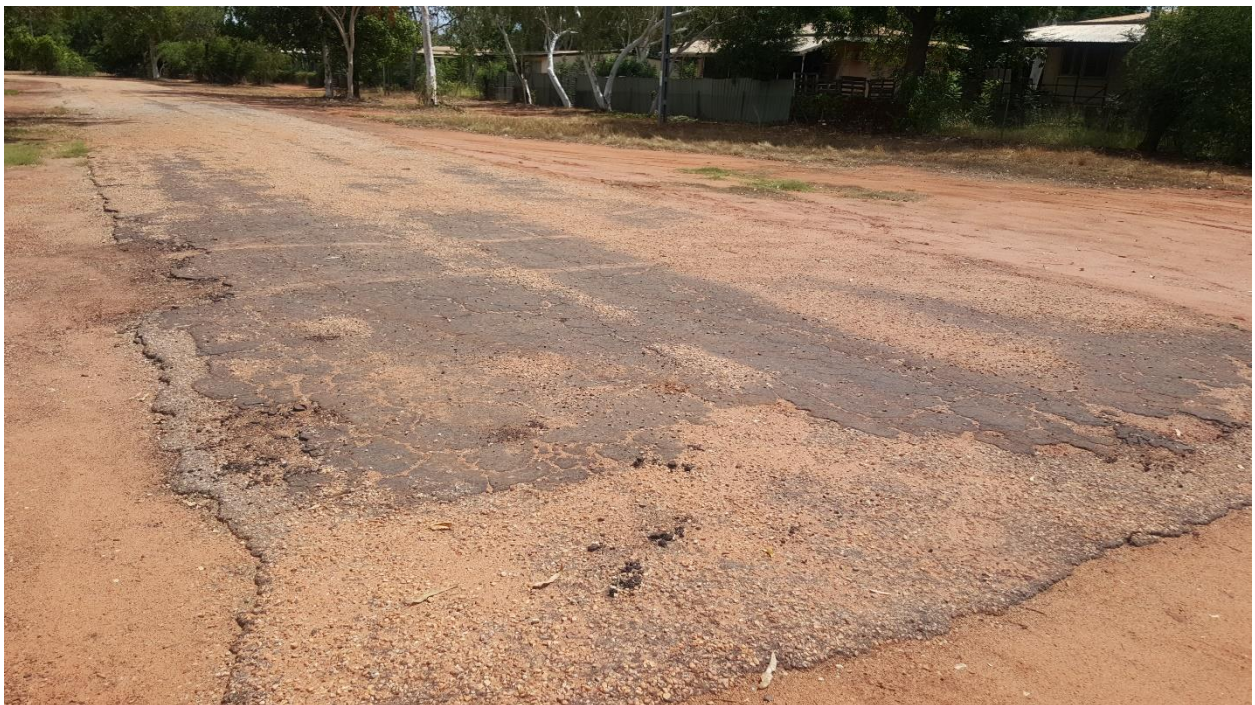
Stripping, Rowell Crt – Condition 5, Very Poor
