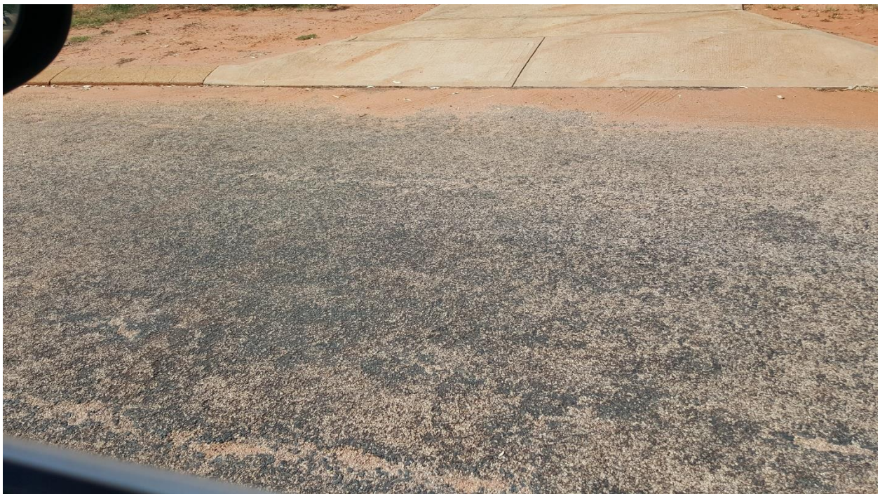
Polishing, Short St – Condition 5, Very Poor
