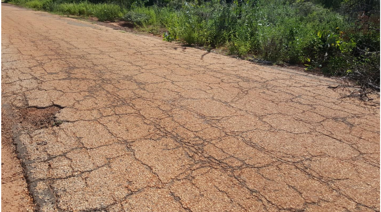
Crocodile Cracking, Granville St – Condition 5, Very Poor
