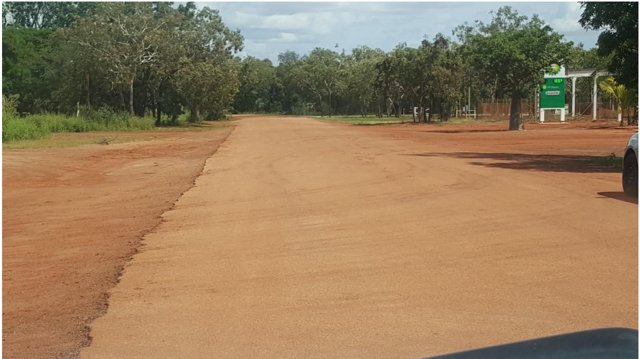
Edge Drop Off, Rodgers St – Condition 4, Poor
