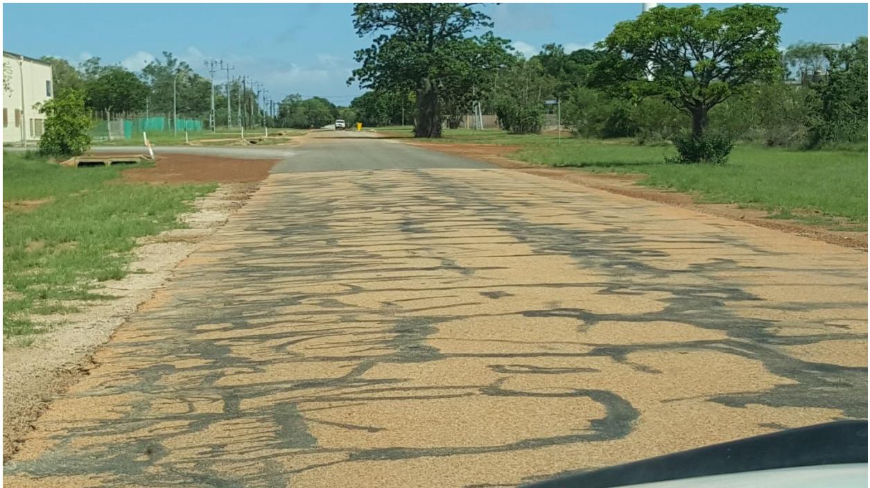
Transverse Cracking, Wodehouse St – Condition 5, Very Poor
