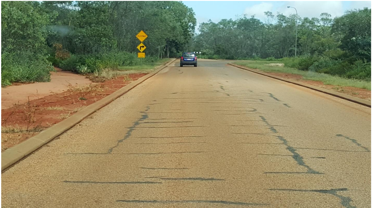
Block Cracking, Fitzroy St – Condition 3, Fair
