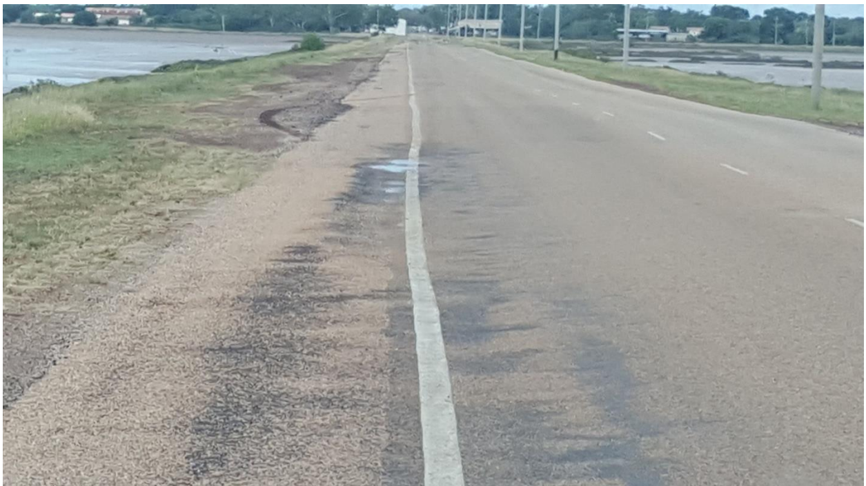
Deformation (rutting), Jetty Rd – Condition 4, Poor
