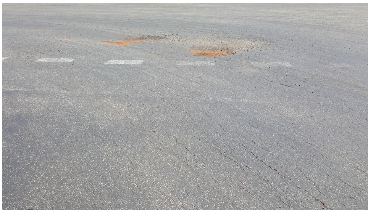
Deformation (shoving), Jetty Access Road – Condition 4, Poor
