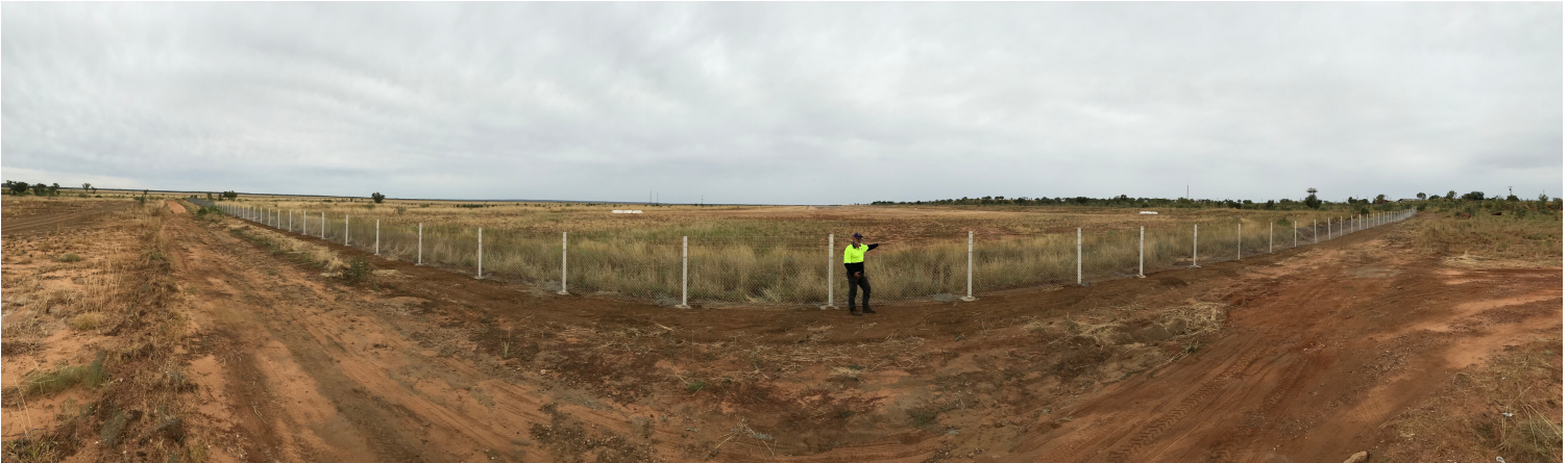
Photo: Cr Geoff Davis surveys the newly installed fencing.
