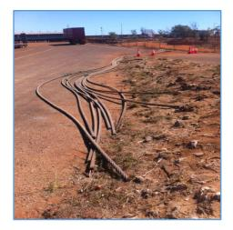
Last week, Mitchell Plastic Welding were also in the car park a rea to construct a number of poly pipes that were each one hundred metres long. With steel cables being inserted into them, they were sealed and towed out to the Marine Produce Australia (MPA) Cone Bay Barra farm.
